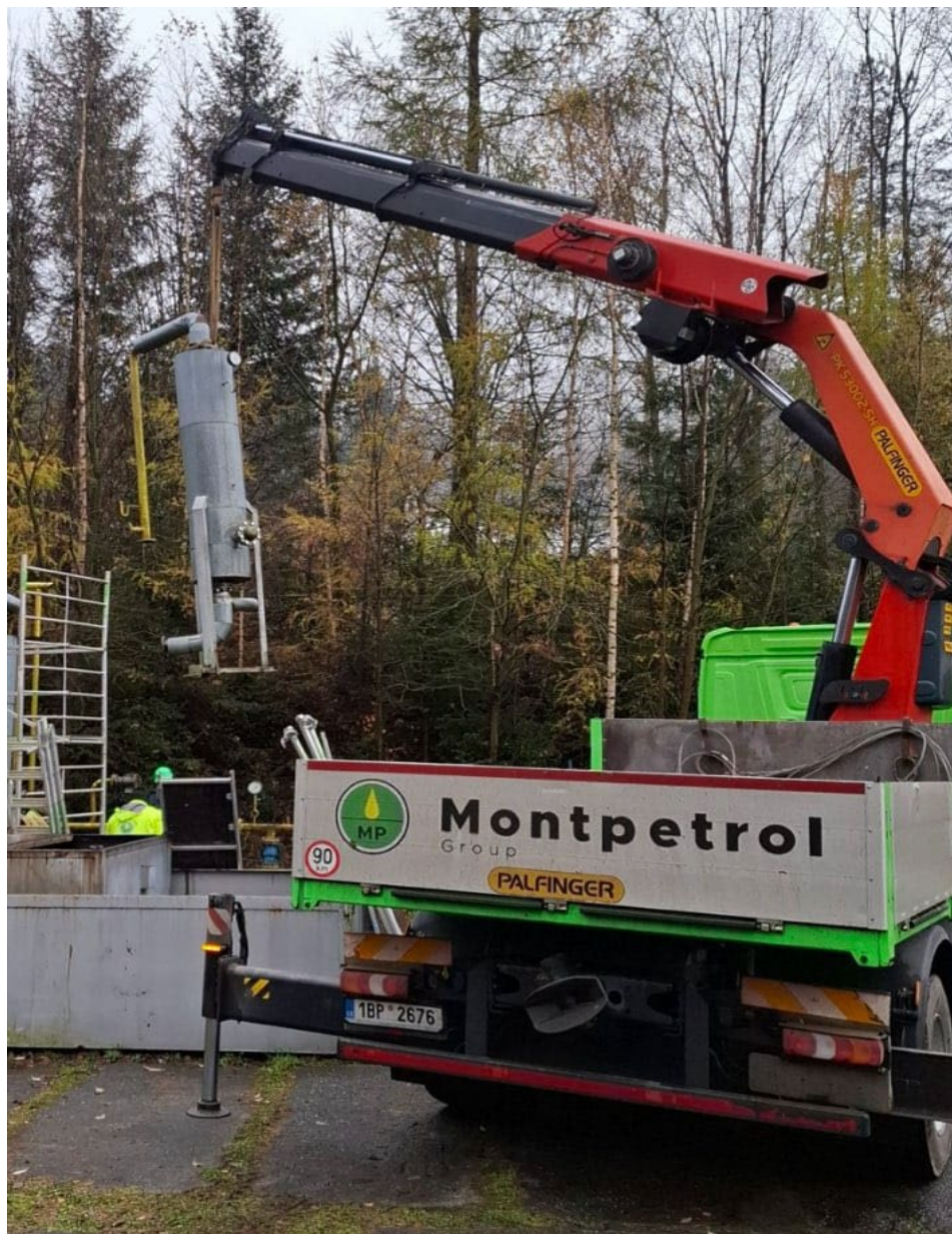
Figure 2 - Moving production equipment onto NP-823
